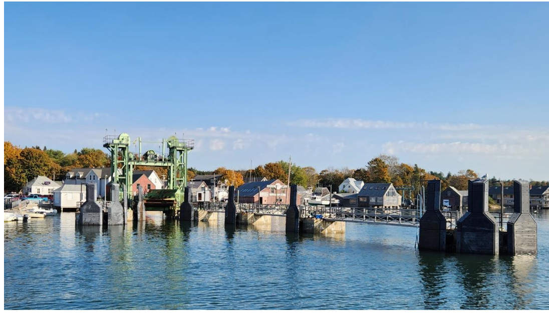
Ferry Terminal NORTH HAVEN, ME
